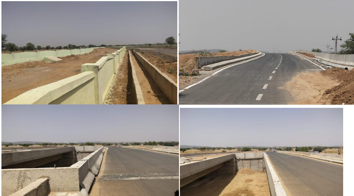
Construction of RCC Storm water drain approaches at I/A Ghiloth.
